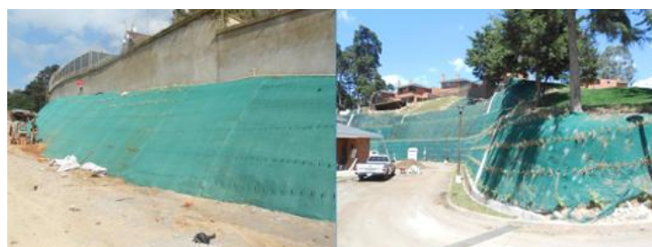
Figure 5 - Photodegradable or Synthetic Geomants. Adapted from Castro (2025).
