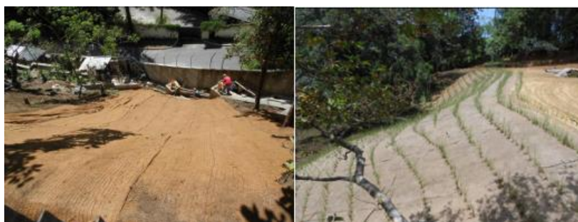
Figure 4 - Biodegradable Geomants. Adapted from Castro (2025).
