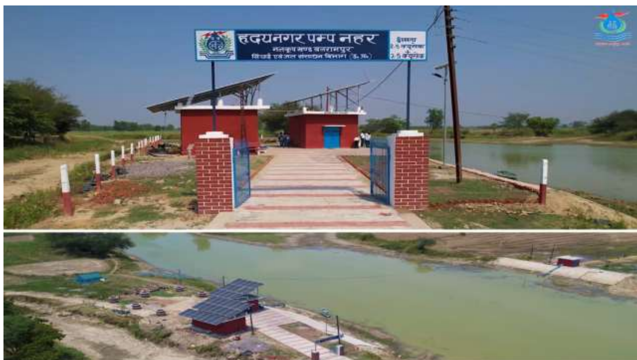
Figure 1. Hriday Nagar Lift Pump Canal Solarisation Actual Site View
