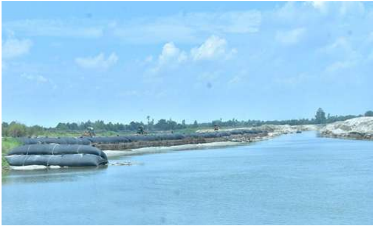
Figure 3. In-situ installation of the three-layer geotube structure for flow diversion
