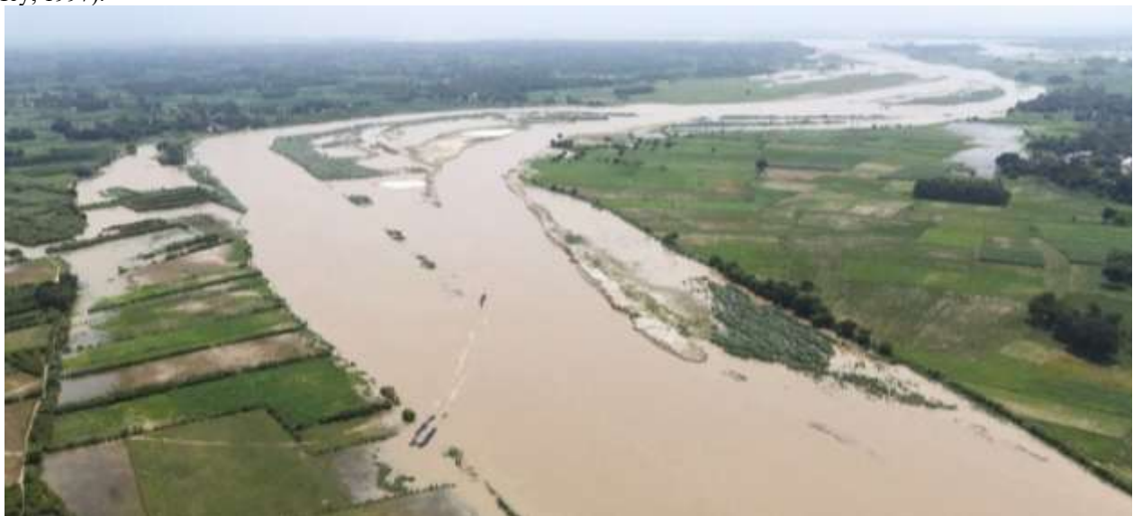
Figure 11. Water flow through dredged channel during monsoon season
