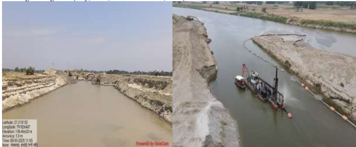
Figure 2. (a) Excavation work by hydraulic excavator (b) Dredging work by dredger
