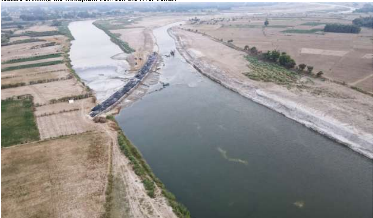
Figure 9. Water flow through dredged channel with geotube diversion
