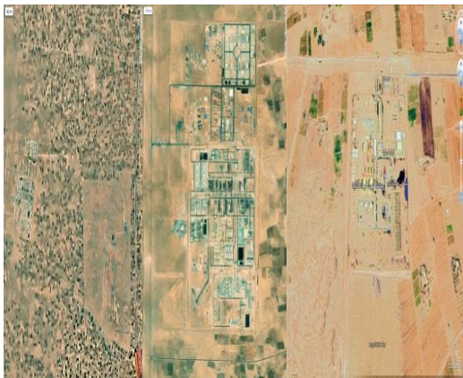
Figure 7: Karbala Airport location, Karbala refinery site and Karbala gas station location
