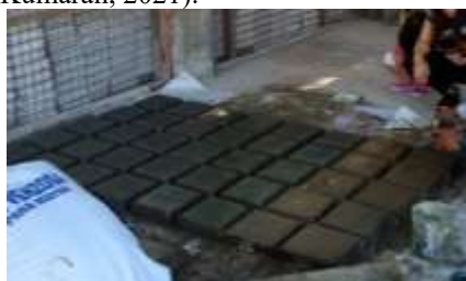
Figure 3. Casting and Curing of Eco-bricks
